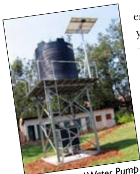
Solar-Powered Water Pump in Uganda
